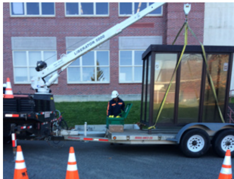
Fairhaven Middle School's WTA shelter is lowered by crane onto its pad.
